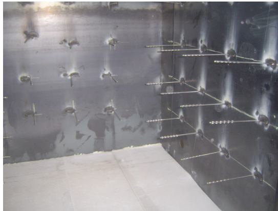
FIGURE 10 – steuds soudés
